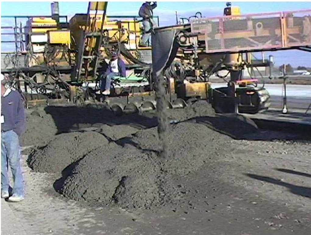
FIGURE 10. TYPICAL PAVING OPERATIONS
