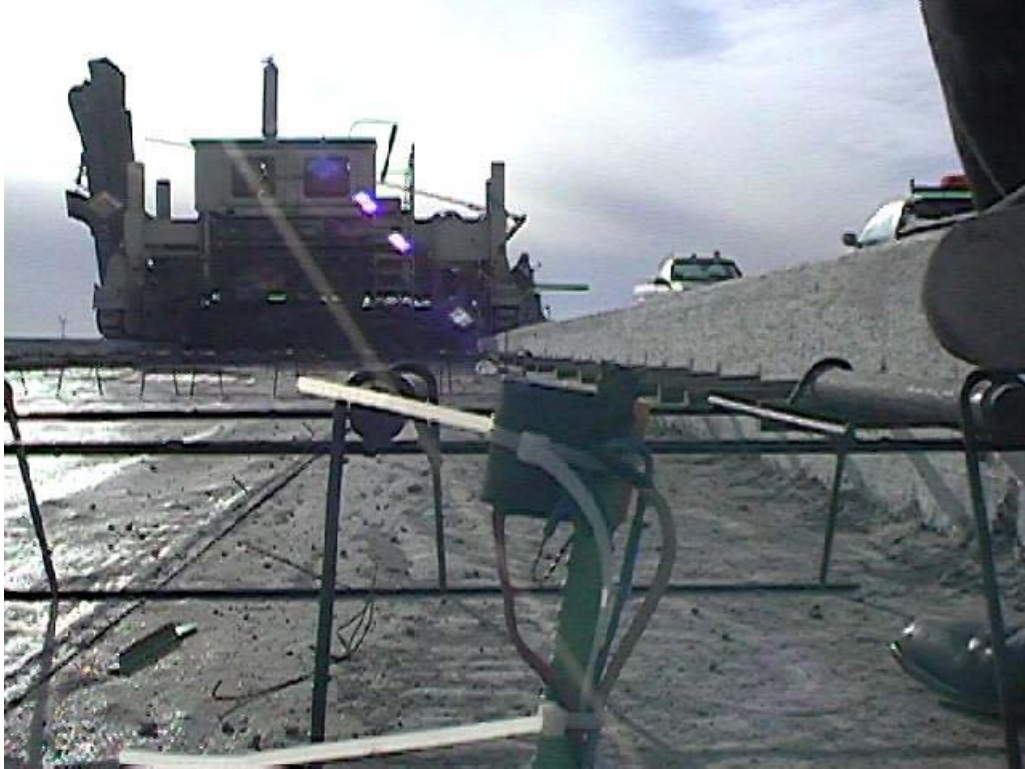
FIGURE 12. MATURITY DEVICES SECURED PRIOR TO PAVING
