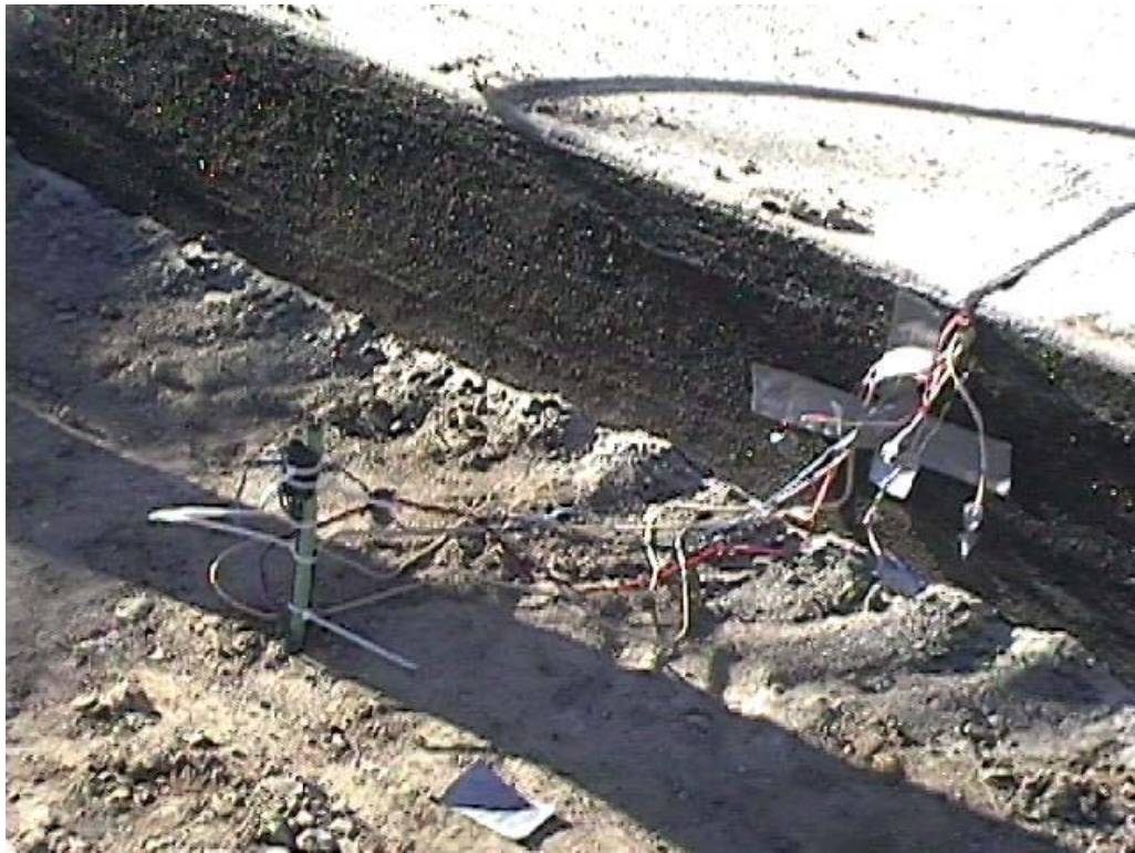
FIGURE 15. SENSOR LEADS SECURED PRIOR TO PLACEMENT
