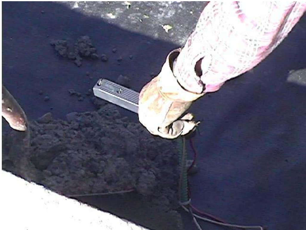
FIGURE 17. CONCRETE SHOVELED AROUND SENSORS TO PROTECT FROM PAVER
