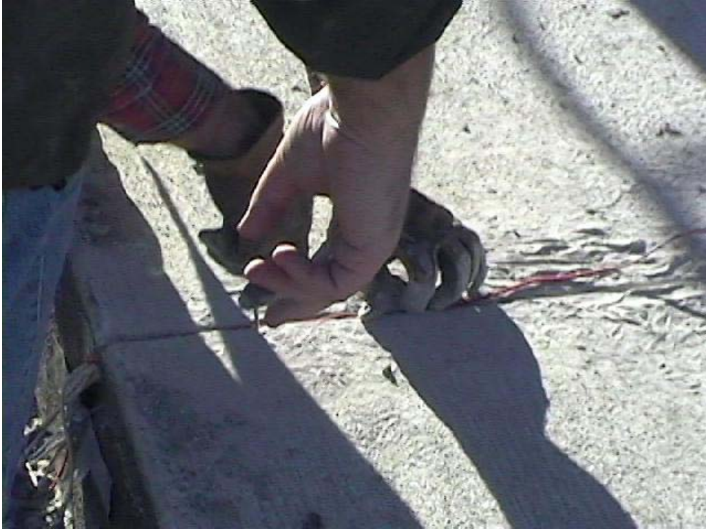
FIGURE 14. INSERTING SENSOR LEADS INTO ADJACENT JOINT CUT
