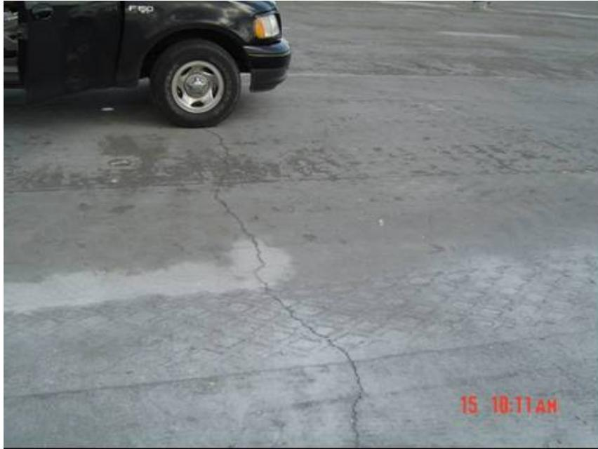
Figure 2-3. Shrinkage cracking in CTB.
