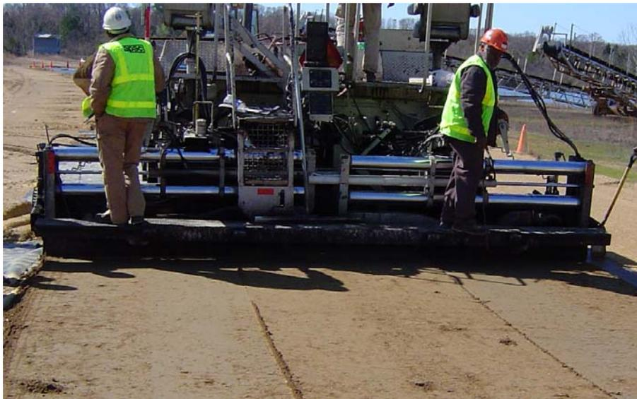
Figure 4-1. CTB placement with an asphalt paver.
