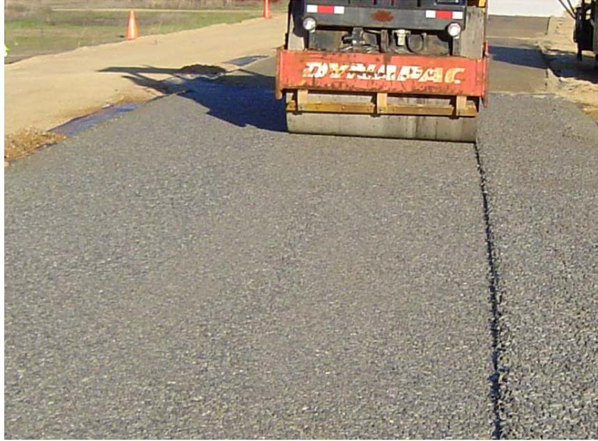
Figure 4-2. CTPB compaction with a static roller.
