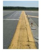
**Holding Position Markings** are positions on or at the movement area where the pilot or surface operator must to stop before getting clearance from Air Traffic Control (ATC) to proceed.
