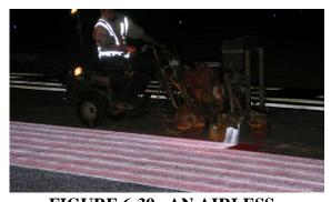
FIGURE 6-39. AN AIRLESS MACHINE WITH A MOTORIZED "SULKY" APPLIES MARKING WITH AUTOMATIC GLASS BEAD GUNS.
