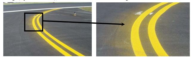
FIGURE 6-44. OVER SPRAY CAUSED BY WIND OR THINNED PAINT, OR BOTH.
