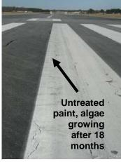
FIGURE 4-18. PAINT USED WAS STANDARD TT-P-1952E.
