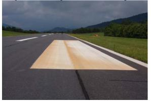
FIGURE 4-24. STAINED LEADING EDGE AND LOW AREA ALONG JOINT WHERE WATER FLOWS.
