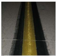
FIGURE 3-9. NON-FUNCTIONAL MARKING DUE TO POOR REFLECTIVTY.
