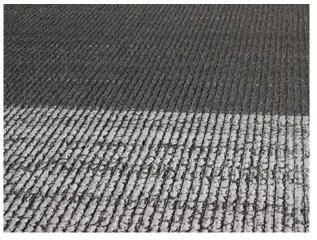
FIGURE 5-22. MARKING BEFORE (BOTTOM) AND AFTER (TOP) REMOVAL.
