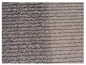
FIGURE 2-6. RESULTS OF WATERBLASTING REMOVAL ON POOR ASPHALT SEEN IN FIGURE 2-5.
