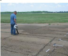
FIGURE 4-39. LEAF BLOWER CLEANS LOOSE RESIDUE AFTER SURFACE PREPARATION.
