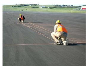
FIGURE 6-3. LAYOUT WITH CHALK LINES ENSURES PROPER PLACEMENT AND ALIGNMENT.
