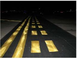
FIGURE 6-35. SIX-MONTH OLD HOLDING POSITION MARKING WHERE BEADS WERE HAND-THROWN.
