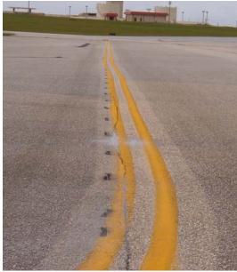
FIGURE 2-4. MARKING IS OUT OF ALIGNMENT
