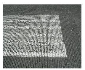
FIGURE 2-5. A PRE-EXISTING CONDITION OF POOR ASPHALT PAVEMENT.
