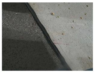
FIGURE 5-14. USED FOR REMOVAL ON NON-GROOVED SURFACES, SHOTBLASTING CAN BE A BEST PRACTICE.
