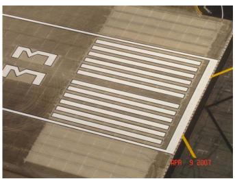
FIGURE 5-33. THE VISIBLE SCAR IS CLEANED PAVEMENT.
