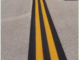
FIGURE 6-43. AIRLESS LINES HAVE SHARPER EDGES.
