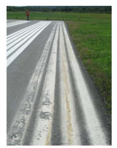
FIGURE 6-16. LAYERED STRIATIONS ON THE SIDELINE WERE SCRAPED OFF BY SNOWPLOWS.
