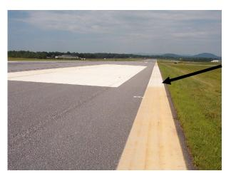
FIGURE 4-25. GROOVED SURFACE MAKES STAIN LESS NOTICEABLE.
