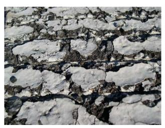
FIGURE 4-5. MAGNIFIED PHOTO OF FIGURE 4-4 SHOWS CRACKED ASPHALT WHERE WATER INVADES.
