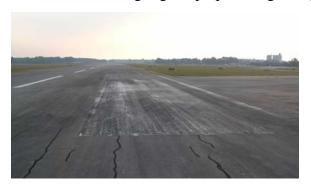
FIGURE 4-16. BEFORE WATERBLASTING: ALGAE OBSCURE MARKING.
