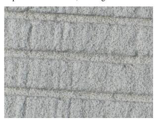
FIGURE 6-5. THE UNPAINTED SIDE OF THE GROOVES IS NOT NOTICEABLE FROM A DISTANCE.
