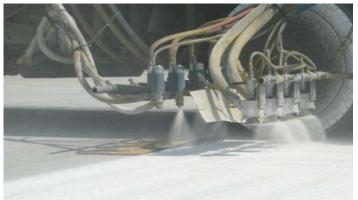
FIGURE 6-28. FOUR PNEUMATIC (ATOMIZED) PAINT GUNS APPLYING A 3-FOOT WIDE PATTERN.
