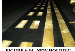
FIGURE 6-34. NEW HOLDING POSITION MARKING WHERE BEADS WERE HAND-THROWN.
