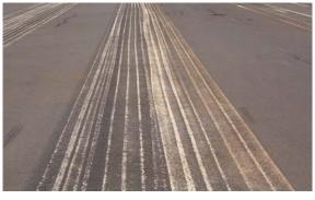
FIGURE 4-2. AFTER CLEANING LOOSE AND POORLY BONDED PAINT BY WATERBLASTING.
