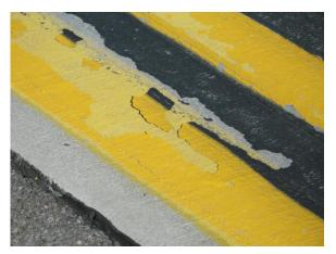
FIGURE 2-1. PEELING PAINT LAYERS
