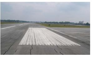
FIGURE 4-17. AFTER WATERBLASTING, BUT BEFORE PAINTING.
