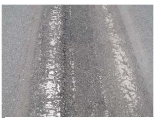
FIGURE 5-30. REMOVAL OF MULTIPLE LAYERS ON DETERIORATED ASPHALT.
