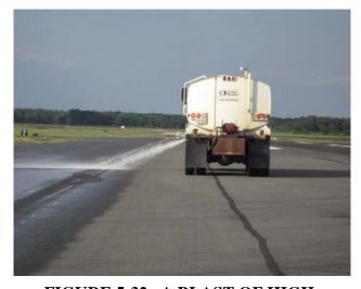
FIGURE 5-32. A BLAST OF HIGH-PRESSURE WATER REMOVES DEBRIS FROM SCAR.
