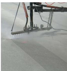
FIGURE 4-38. LOW-PRESSURE WATERBLASTER.
