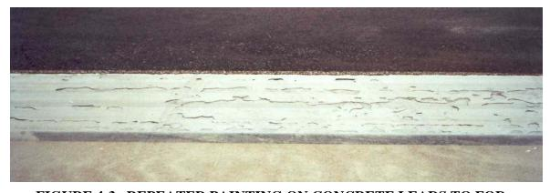
FIGURE 4-3. REPEATED PAINTING ON CONCRETE LEADS TO FOD.
