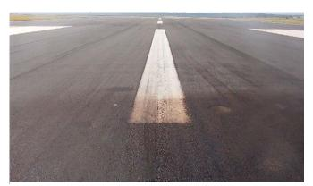
FIGURE 4-32. THE OILY STAIN WILL PREVENT NEW COATING FROM BONDING.
