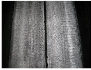
FIGURE 4-40. HEAVY RUBBER DEPOSITS WERE REMOVED FROM THIS CENTERLINE MARKING WITH ULTRA HIGH-PRESSURE WATERBLASTING.
