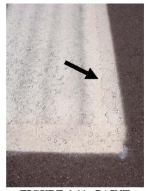
FIGURE 4-11. PAINT CRACKS WHEN APPLIED TOO THICKLY.
