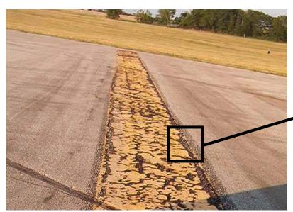
FIGURE 6-10. OLD SOLVENT PAINT CURLED, CRACKING THE ASPHALT TO WHICH IT WAS BONDED.
