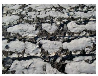
FIGURE 5-23. EVIDENCE OF BOTH PAINT AND ASPHALT CRACKING INDICATES PRE-EXISTING CONDITION.
