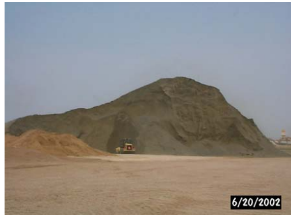
Figure 6.3 – An excessively high stockpile
