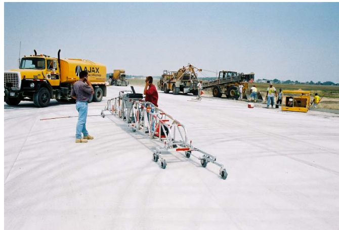
Figure 10.4 – Profilograph testing in progress
