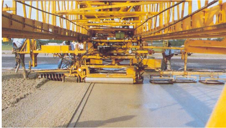
Figure 8.1 – Typical bridge deck paving operation
