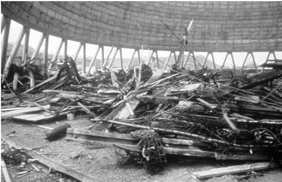
Figure 3.3 – Portion of the Willow Island Cooling Tower Collapse (source: <http://www.geocities.com/pburgwva2001/willow1.html>)
