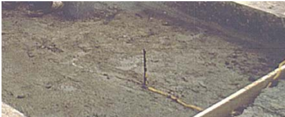
Figure A.9 - Temperature Sensor in Concrete Pavement Repair Area
